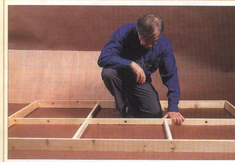
Begin by identifying the parts. There are three 6ft timbers and four 4ft pieces. These all have cross-halving joints cut in them. The 3in deep pieces form the front, back and sides of the frame while the 2in pieces are the inter-locking cross-braces.
